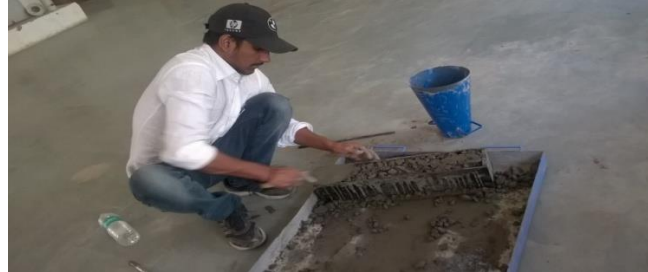
Fig. 1: Casting of Beam
