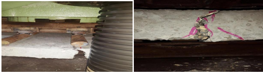
(a) Without steel fiber (b) With steel fiber Figure (7) Failure in flexural steel fiber concrete slab (a) without steel fiber (b) with steel fiber
