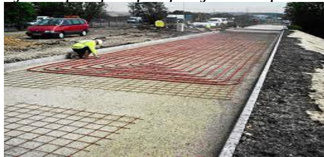
Figure. 3 Pipes in form of Reinforce grid to avoid peak stress.
