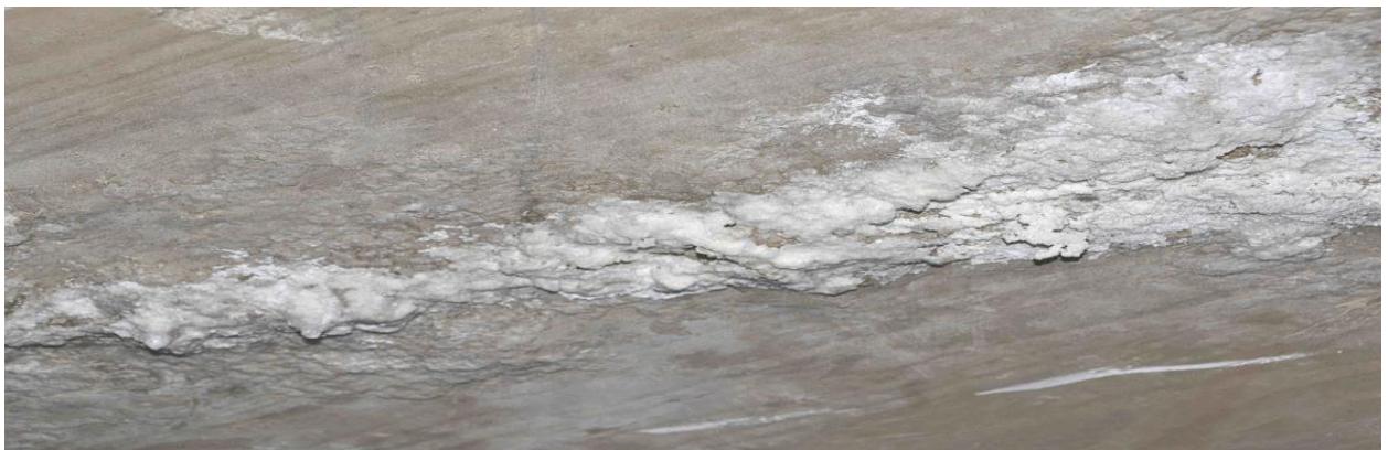
Fig 2 : Example of secondary efflorescence in parking garage exposed to diluted road salt from vehicles entering the garage during winter.
